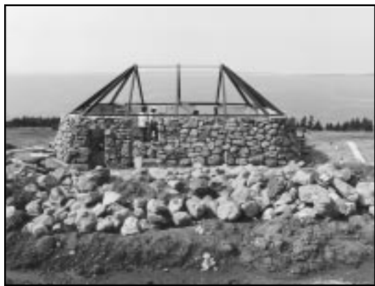
Construction of the MacCallum House, blackhouse in 1995.
