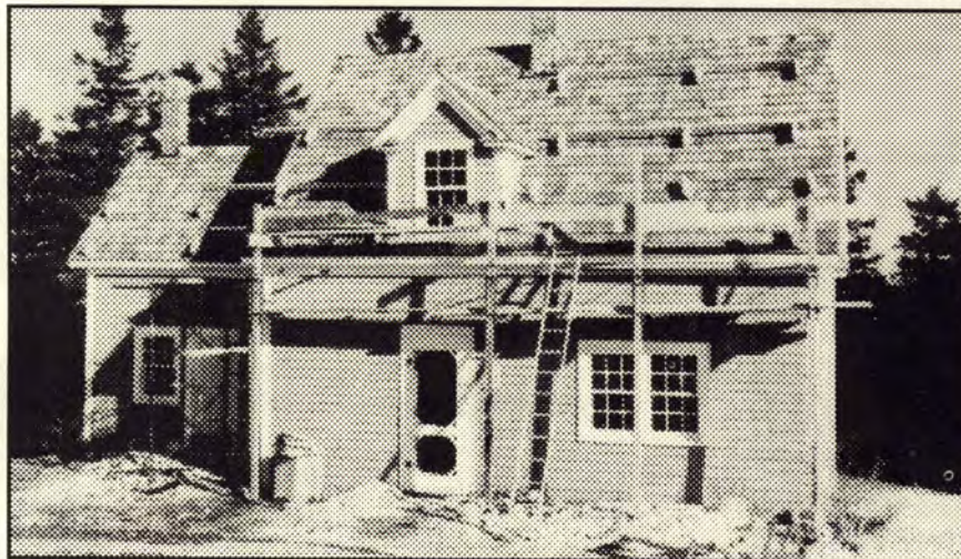
Working on the 1900's roof.
