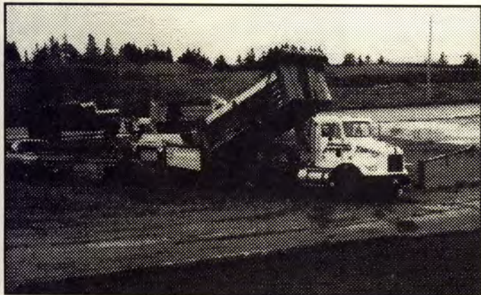
Here comes the asphalt.
