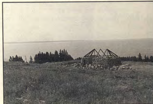
Preparing for the roof of our new blackhouse.
