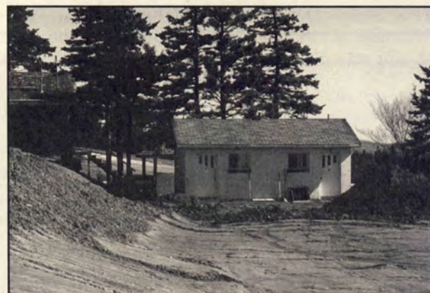
Construction of the new expanded and paved parking lot.
