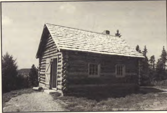
Exterior of the MacEachern Log Dwelling (taken en route from the Blackhouse).
