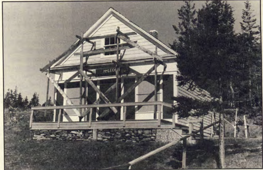
Construction work on the front of the General Store.
