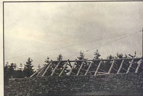
Preparing for the roof of our first blackhouse.
