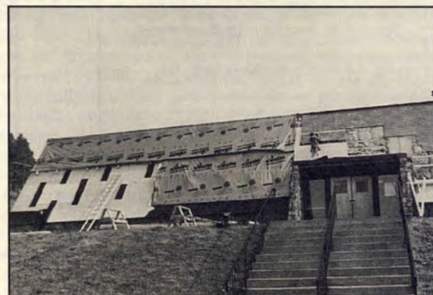
Renovation work on the Visitor Centre
