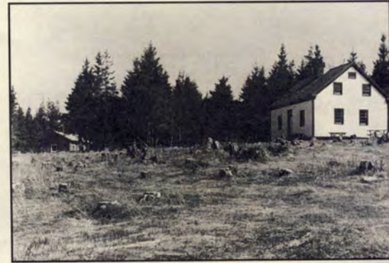
Land being cleared between the MacDonald House and Barn.
