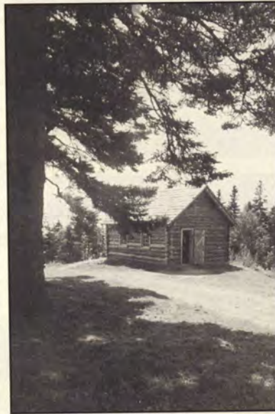
Exterior of MacEachern House through the woods from the MacDonal House.
