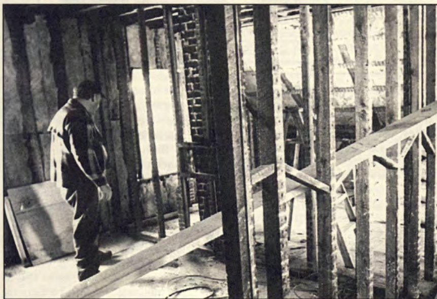
Hector MacKenzie working on the interior restoration of the MacQuarrie-Fox House.
